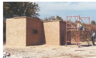
**Structures made with Grancrete can withstand extreme temperatures without cracking, and are termite and vermin proof.**
