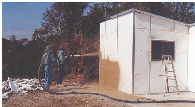
**Grancrete, a sprayable, concrete-like product, can be sprayed over a wide variety of surfaces, making them waterproof and fire-resistant, according to the manufacturer.**
