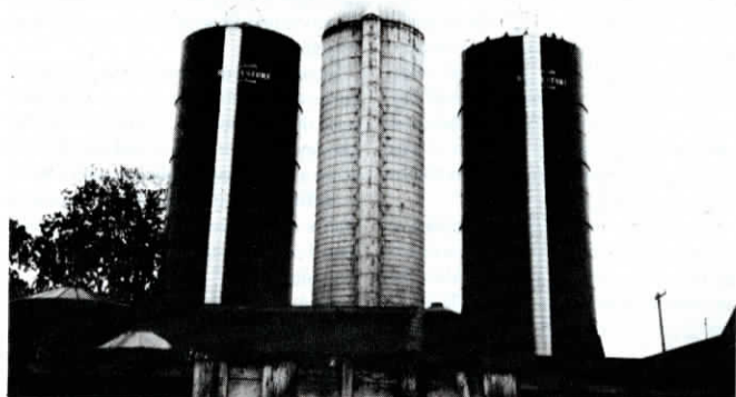
Jim Beckham added doors, chutes, and top unloaders to these Harvestore silos.
