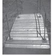
Miles Aronson says working with Quonset sections is easier than working with raw corrugated metal. Predrilled holes make it easy to bolt sections together and add half sections to the sides to make the bridge wider.
