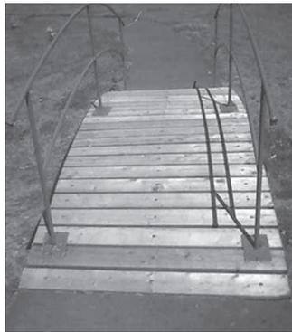
Miles Aronson says working with Quonset sections is easier than working with raw corrugated metal. Predrilled holes make it easy to bolt sections together and add half sections to the sides to make the bridge wider.
