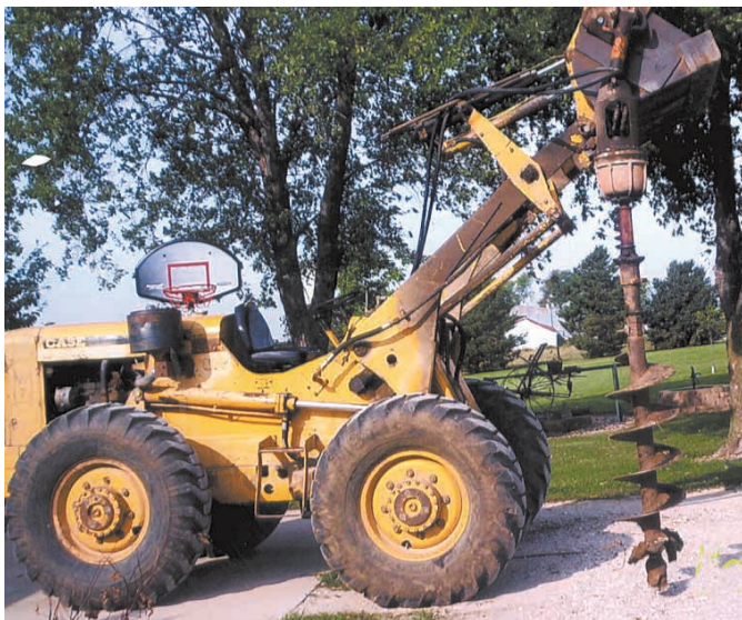
Mounted on a used payloader, auger is 18 in. in dia. and will dig 8 ft. deep. Boling uses it to set 12-ft. long corner posts in the ground.
