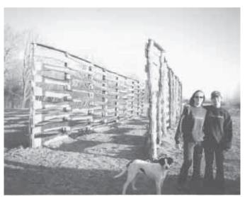
Perry Bubnick designed this 50-cord "air dryer" by setting up two 80-ft. long rows of 10-ft. tall poles, spaced 8 ft. apart. He nailed 1-in. thick oak slabs to the inside.
