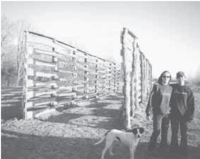
Perry Bubnick designed this 50-cord "air dryer" by setting up two 80-ft. long rows of 10-ft. tall poles, spaced 8 ft. apart. He nailed 1-in. thick oak slabs to the inside.
