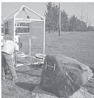
Boulder-building process uses concrete and additional additives that strengthen and prevent water penetration.
