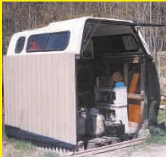
to the outside of the skids and added some caulk to make the shelter water-tight. By setting the walls on a 2 by 6 bottom plate, I can use a truck or tractor to tow the building to a new location. (Louis Trepanier, Rt. 2, Haliburton, Ontario, Canada K0M 1S0)
