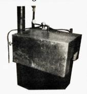
iron radiators for the grates. It has an ash pan about  $3\frac{1}{2}$  in. deep that needs emptying once a week. There is a  $210^\circ$  pop-off valve on top, along with a temperature guage.
