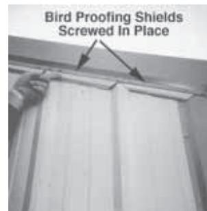
**Bird-proofing shields screw in place over ventilation gaps between sidewalls and roof.**
