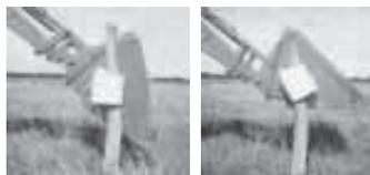
**Operator slips pipe over post, tilts bucket up at an angle so the teeth grip the post, and then raises loader to lift post out of ground.**
