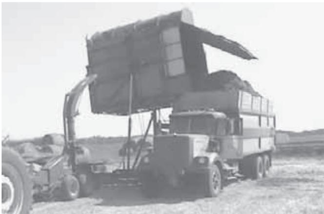
Palechek placed stackwagon box on end, with floor bottom toward tipping side of wagon. Box is hydraulically raised and tipped on its side to load truck.
