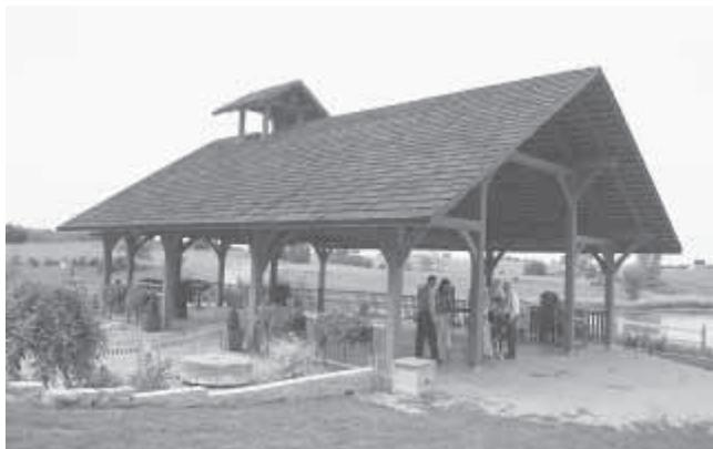
Post and beam shelter provides a place to go when the weather does not cooperate. The Nortons built it from scratch, using timbers from old barns and grain elevators.
