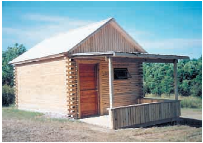
Clyde Barnhart uses landscape timbers to put up buildings that have a "log cabin" look to them.
