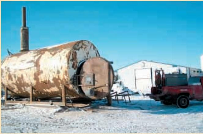
Large capacity bale furnace heats 40,000 sq. ft. at a fraction of the price of LP gas.
