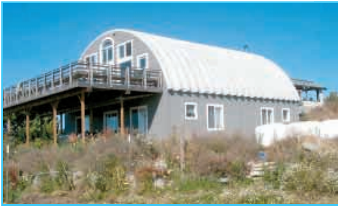
Skip Clark used a 40 by 40-ft. quonset building to cover the top floor of his new two-story house. Both ends of the upper floor are virtually all glass.
