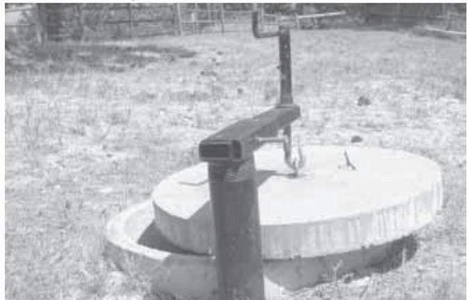
Horizontal bar with a crank shaft on the end is used to lift cover off septic tank.
