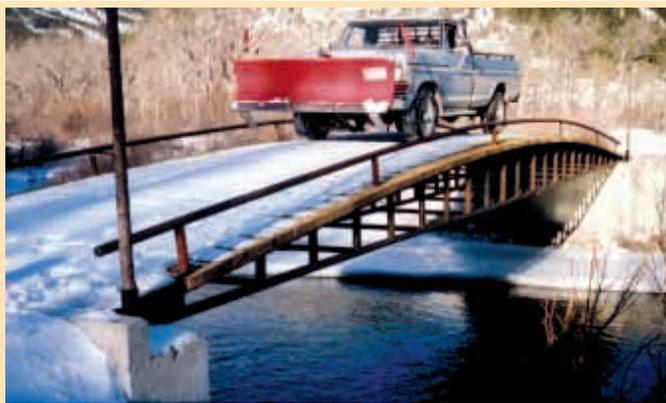
To build vehicle bridges, Ed Stahler uses two spans with bridge planks over top for a 10 to 12-ton load rating.
