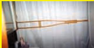
I'm 78 years old and I sometimes get dizzy in the shower. So I came up with the idea of a guard rail made out of an old crutch. I put a couple nails in the shower wall frame and drilled holes in either end of the crutch. So it's easy to set the crutch in place and take it down. Since crutches are made from hard wood, they're very strong and will easily support my weight if I should need it. (Merrill Ray Kopp, Shady Spring, West Virginia)
