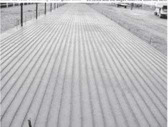
Concrete "groover" lets you make grooves in a freshly poured concrete floor to provide
