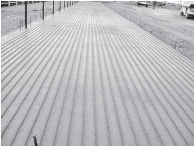
Concrete "groover" lets you make grooves in a freshly poured concrete floor to provide better footing for livestock.
