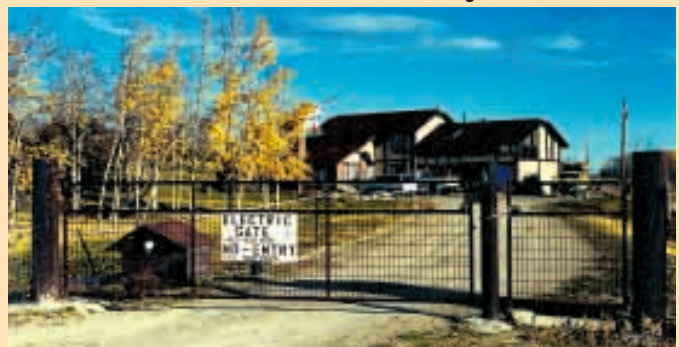
Remote-controlled security gate was made from a garage door opener and doorbell.
