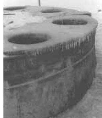
McCoy made two 2,500-gal. freeze-proof cattle waterers by cutting a 5,000-gal. fuel tank in half and burying the two halves "standing up" in the ground.
