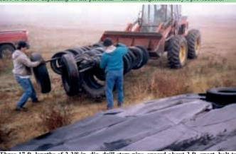
Three 17-ft. lengths of 2 3/8-in. dia. drill stem pipe, spaced about 3 ft. apart, bolt to bucket. Pipes carry about 50 car and truck tires at once.
