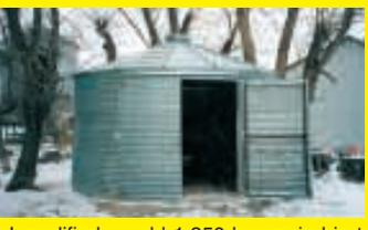
I modified an old 1,350-bu. grain bin to store wood for my outdoor furnace. I cut out a pair of doors that measure 6 ft. 4 in. wide. I used 2-in. wide, 5/32-in. thick
