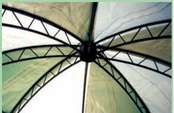
Secret to design of new domed building is the new center hub which joins conventional hoop-type trusses together.
