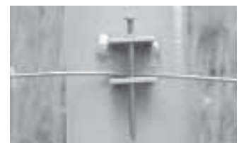
Example of a welded-on steel post clip.
