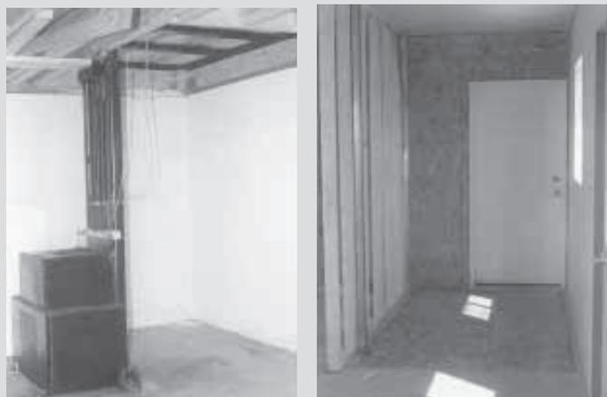
Homemade elevator was built out of a salvaged forklift mast (left). When the elevator is down (right), floor is level and the family walks right over the top of it.
