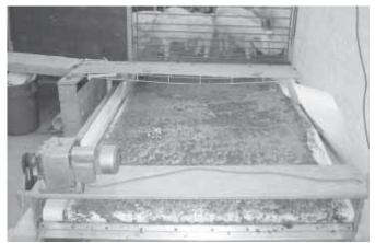
Conveyor belt runs length of barn beneath slatted portion of pens, moving manure out of barn. Belt is tilted at a 4 degree angle, so urine runs into channel along lower side.
