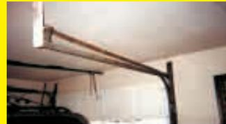
On my door, the springs ran alongside the door. The problem is that if the spring breaks, it comes free with great force, which can be dangerous and damage vehicles. I solved the problem by running a wire through the center of the spring and anchoring the wire securely at either end. That way, if the spring breaks, it can't go anywhere. **(John Graham, 8022 Kraft Ave. S.E., Caledonia, Mich. 49316)**
