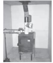
Measuring 20 in. wide, 24 in. deep, and 25 in. high, boiler handles 18-in. logs.
