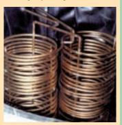
Tank contains two heat exchange coils connected in parallel. One set of coils heats water in the tank. The other set picks up heat from the tank to carry into the house.
