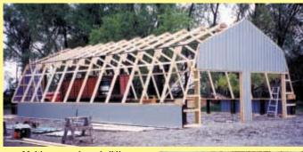
Multi-purpose hoop buildings are made of wooden 2 by 6's with slots cut into them where pipes are inserted lengthwise down the building (a bove). The canvas touches only the pipes, not the wood corners, so there's no wear. You end up with a metal clad building with a silver tarp, at a fraction of the cost of conventional storage sheds.
