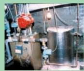
To build his own hot water heater, Marion Palmer bought a polypropylene high temperature tank that's designed to withstand 200-degree temperatures.
