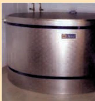
Wood-fired furnace heats water in a large insulated water tank. It stores the heated water until it’s needed to heat the house or shop. It lets you run your wood furnace at full capacity and capture all the heat.
