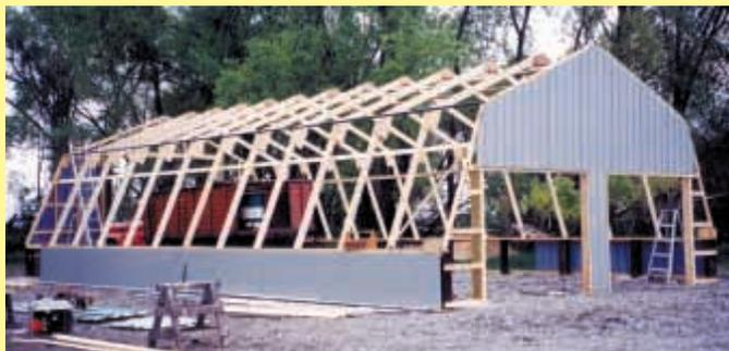
Multi-purpose hoop buildings are made of wooden 2 by 6’s with slots cut into them where pipes are inserted lengthwise down the building (above). The canvas touches only the pipes, not the wood corners, so there’s no wear. You end up with a metal clad building with a silver tarp, at a fraction of the cost of conventional storage sheds.
