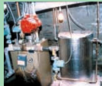
To build his own hot water heater, Mahlon Palmer bought a polypropylene high temperature tank that’s designed to withstand 200-degree temperatures.
