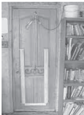
Water bottle is tied by rope to a sliding door. When bottle fills up, gravity pulls it down, opening the door and allowing Fink's dog to go outside.
