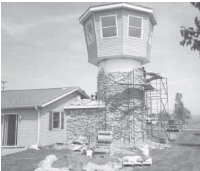
Mark Friebe built this airplane hangar and octagon-shaped air traffic control tower in his back yard. Tower is 30 ft. high and is covered with slabs of native limestone.
