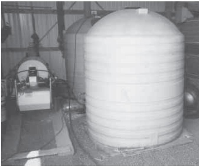
Albert Thiessen uses a sump pump to transfer collected rain water through an underground line into two 500-gal. plastic tanks, located inside his machine shed.
