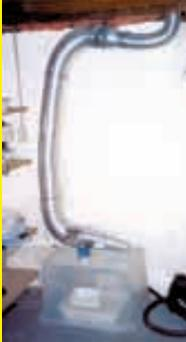
a vent installed next to the clothes dryer vent. An in-line electric fan mounts inside the ductwork and is activated by a motion detector on top of the box. The fan connects to a 20-minute timer. The cat enters the box through a hole in one side, which starts up the fan. It stays on for 20 minutes.
