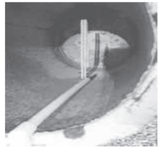
Heater's original element was replaced with a 4,500-watt element. Thermostat's bulb sensor is protected by a section of PVC pipe added inside the tank.
