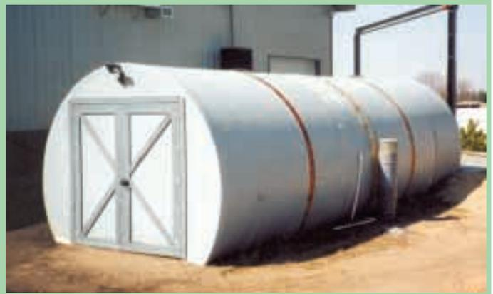
Jim Kaczmarek used a pair of 15-ft. long, 12-ft. dia. fiberglass tanks to make this storage shed that's located next to his shop. He cut off one end of each tank and then placed them together end to end.
