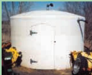
The end of one 12-ft. dia. tank is used to store old tires. It has a door on one side and an asphalt floor.
