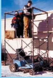
Once the mobile scaffold is in position, stabilizer feet are dropped to the ground to hold it as securely as any other scaffold.
