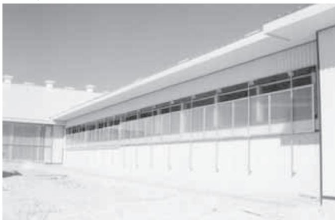
Nova Lite drop panels are made with same kind of unbreakable polycarbonate glass used in greenhouses. Even when they're closed, natural light can still enter building.
