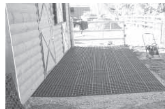
Thin layer of topsoil is placed on top of interlocking grids.
