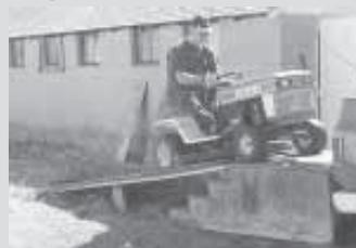
**Bill and C.F. Marley, Nokomis, Ill.:** "A set of ready-made concrete house steps serves a double purpose as a platform for a light-weight ramp and a nice work surface for jobs just outside our shop. The ramp is 12 ft. long and is made from double sheets of plywood mounted on top of 2 by 4 rails. There's a supporting bridge midway up the ramp."
