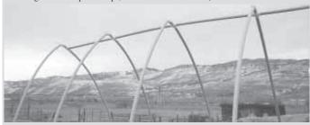
PVC pipes stand on lengths of steel rerod stuck in the ground.
