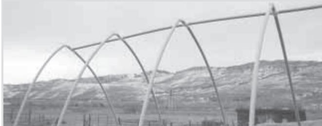
**PVC pipes stand on lengths of steel rerod stuck in the ground.**
