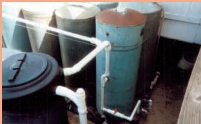
From the gutters, rainwater runs into eight interconnected 120-gal. storage tanks.
