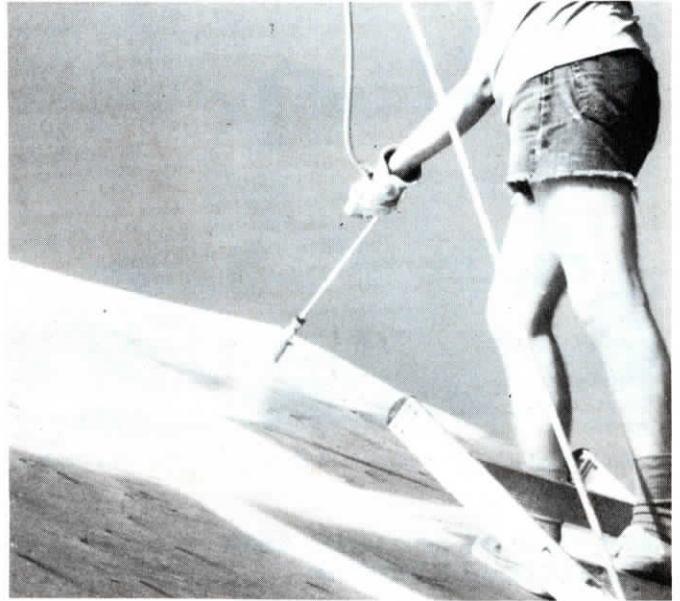
Rapid Roof can also be sprayed on. Conklin offers special Rust Not coating for use on badly rusted metal roofing or siding.
