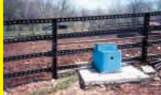
rails used for suspensions on semi trucks. These 16-ft. lengths of rail can be easily formed together to make large corrals. I drive shorter pieces of rail 3 1/2 ft. into the ground about 8 ft. apart. I use four rails per section, which allows the fence to be 5 1/2 ft. high. Because of the holes in the "J" iron, it is easy to mount gates and other equipment. The best part is that it is all salvaged material and cost me cents on the dollar. **(Jim Horn, 379 Gentry Rd., Seymour, Mo. 65746)**
