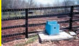
rails used for suspensions on semi trucks. These 16-ft. lengths of rail can be easily formed together to make large corrals. I drive shorter pieces of rail 3 1/2 ft. into the ground about 8 ft. apart. I use four rails per section, which allows the fence to be 5 1/2 ft. high. Because of the holes in the "J" iron, it is easy to mount gates and other equipment. The best part is that it is all salvaged material and cost me cents on the dollar. **(Jim Horn, 379 Gentry Rd., Seymour, Mo. 65746)**
